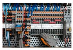
The switch cabinet of the wire rope hoist has a modular design: all components are plug-and-play and can be purchased on the open market from the production of well-known manufacturers - a huge service advantage!
